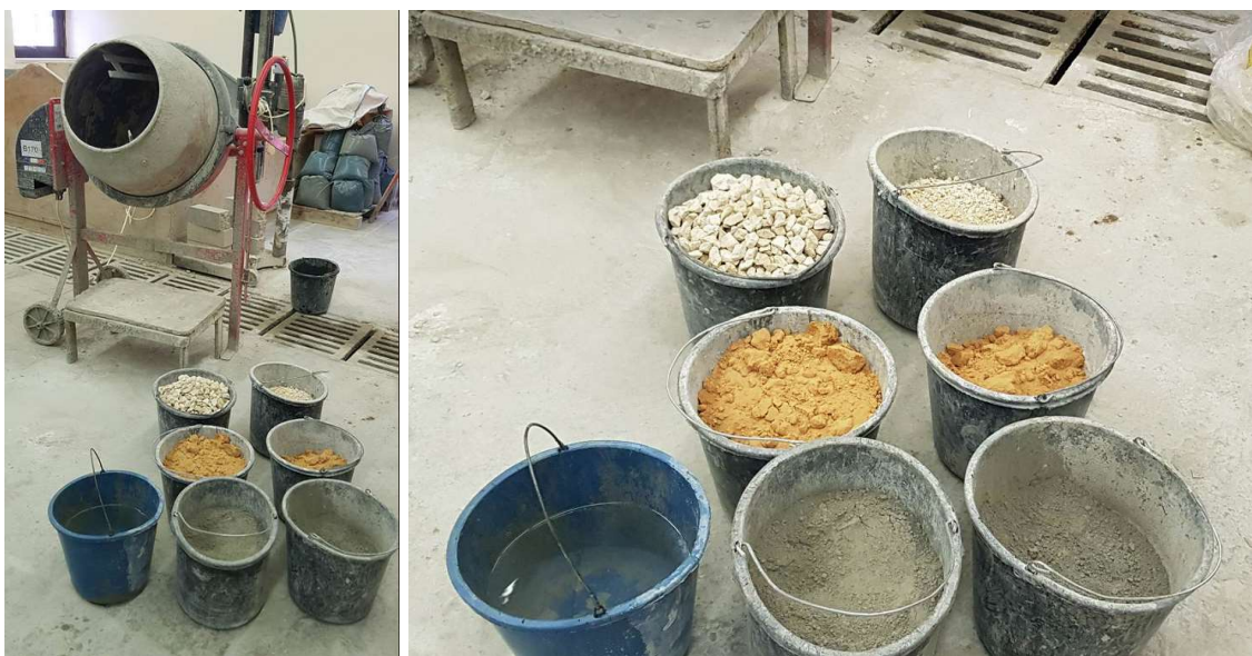
Figure 11: Concrete mix material preparation for mixing.
